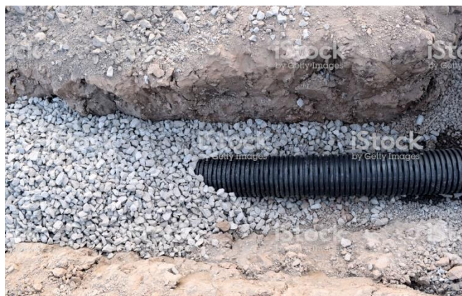
Gravel-packed Sewer Line
