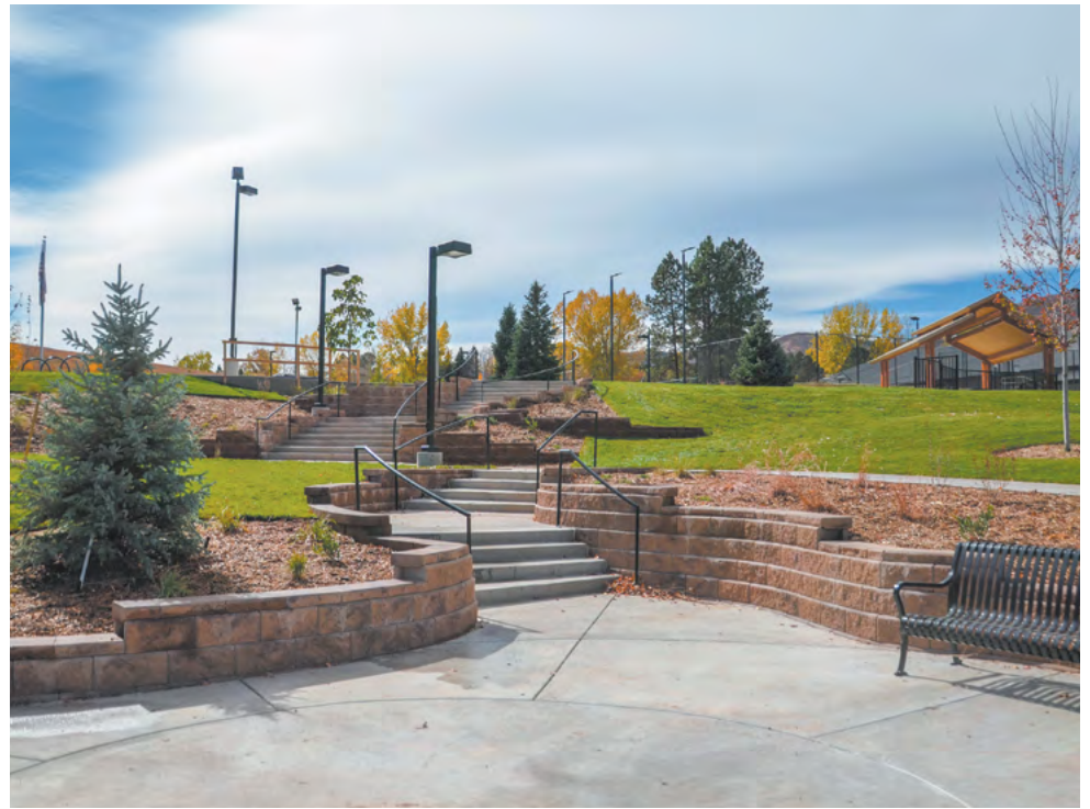
The Community Center site work is now finished, and it features beautiful landscaping, pathways and better access to the facilities.
