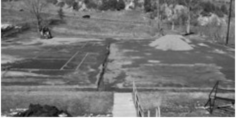
Community Center: The new post-tension tennis courts will be built directly on top of the previous asphalt courts providing a suitable surface from which to build.
