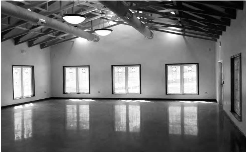
The Lodge Room addition at Dakota Lodge adds approximately 1,650 square feet of multi-purpose rental space to the building.
