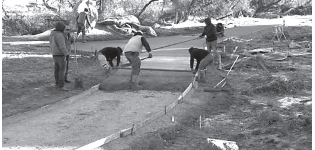
Workers spread wet concrete and apply finish.
