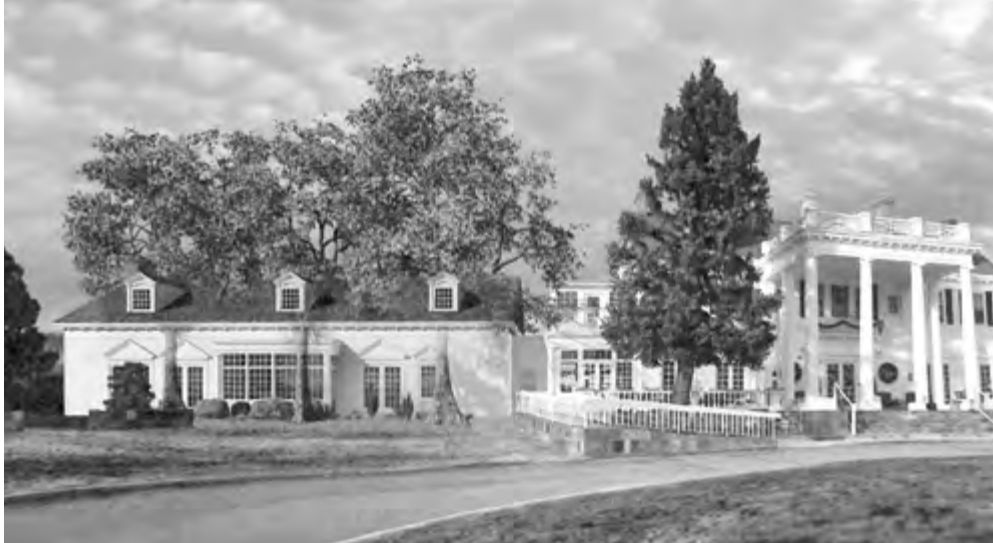
The Manor House addition, shown here, should be completed by early June.
