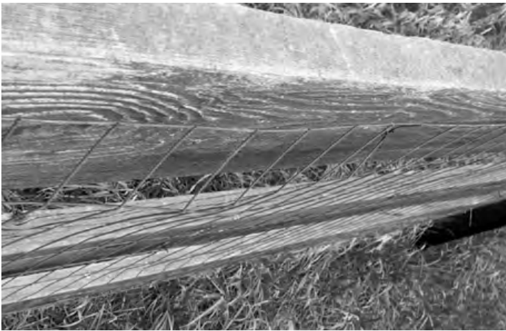
Welded wire should be attached to split-rail fences with staples or U nails.
