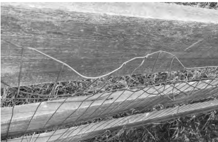
This photo shows welded wire that is not properly attached to the fence, putting deer at risk.
