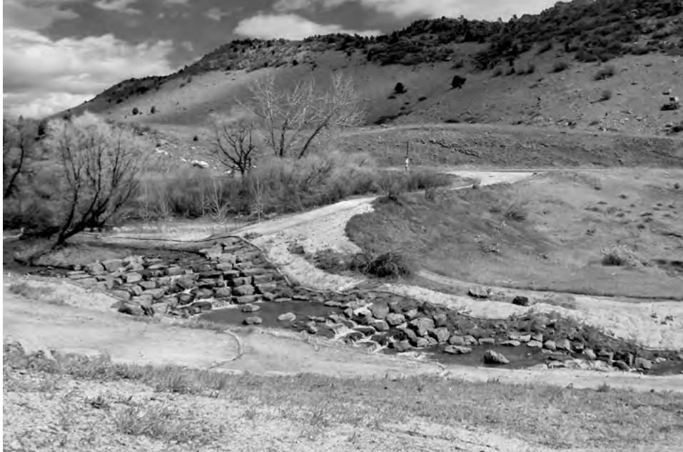
The drainageway improvement project on Massey Draw along the east side of the Community Center is now complete.
