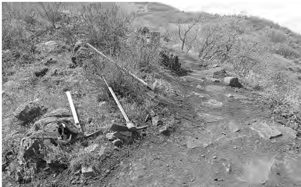
Trail Armoring on Cougar Trail, Credit: Aaron Cholewa (Singletrack Trails, Inc)
