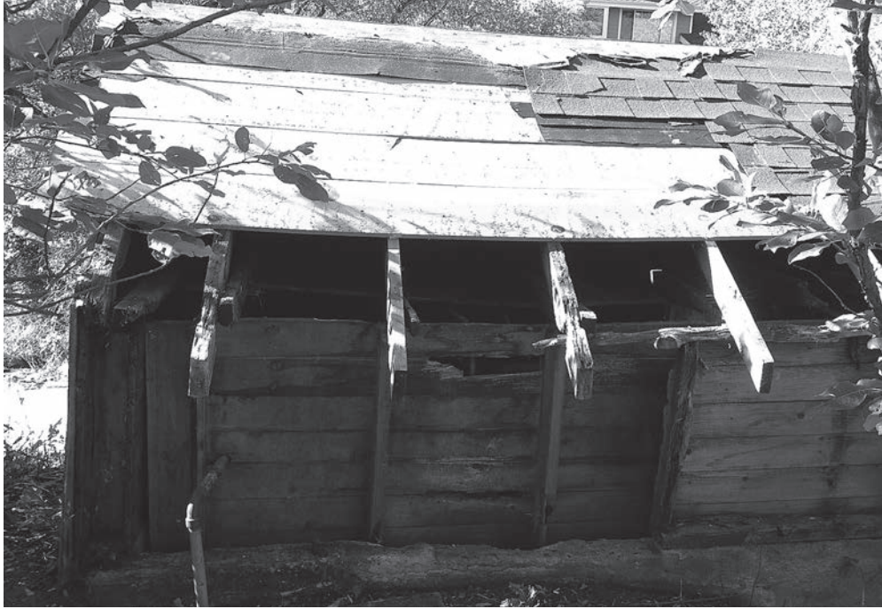
Pump House before renovations.
