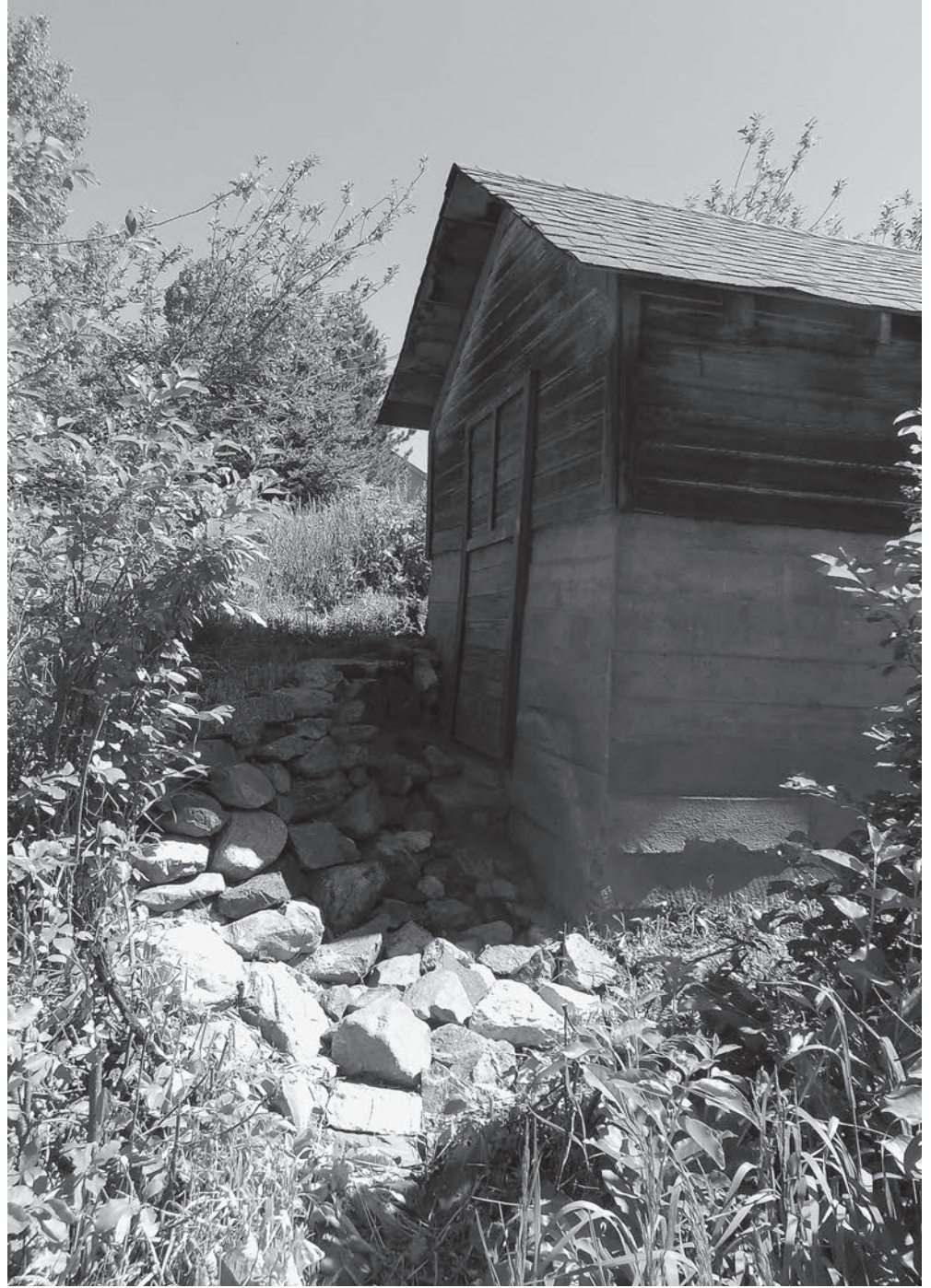
Pump House after renovations.
