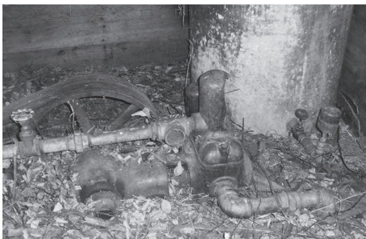
Condition of the actual pump found inside the building before renovations.
