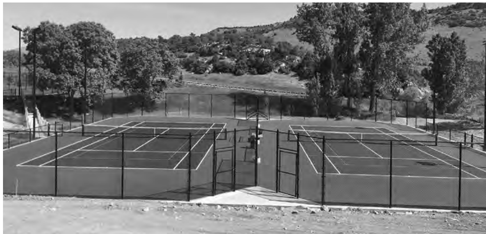
The new post-tension tennis courts at the Community Center are ready for use.
