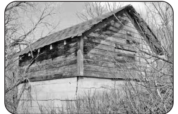
Pump House on Massey Draw
