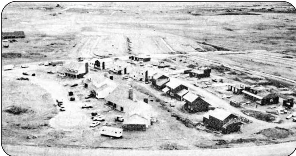
Construction at Quail Ridge, 1976
