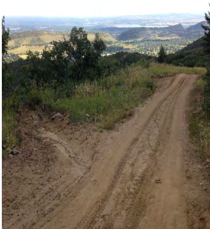
Manor House trail/road, showing turnouts to remove water from road surfaces.
