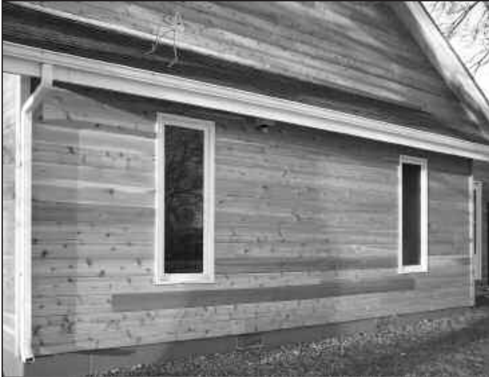
Sections of the siding and front of the Ranch House were deteriorating, and the Master Association recently hired a contractor to replace the wood. The total cost of the project was around $11,000. Some of the wood was original to the Ranch House, which was built in 1975. Due to exposure to the elements, the wood was splintering, cracking and rotting.
