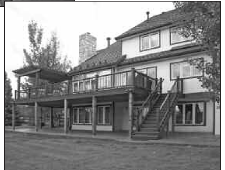
Maverick can design and construct custom decks for your backyard.
