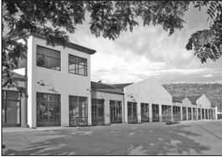
GarageTown's all new Select-Flex units offer glass storefronts, windows, extra parking and opportunities for signs.
