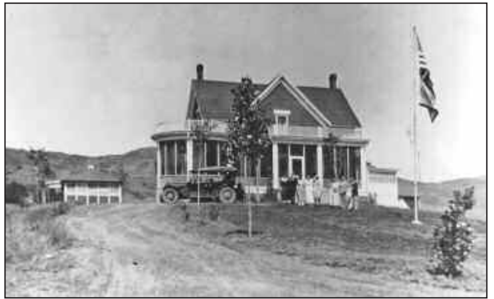
Carroll's House is no longer standing, but evidence of the stone foundation can be picked out among the grasses near the Stone Bridge near Woodruff Drive.
