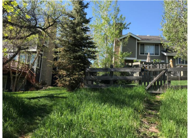
Photo 7: Un-pruned conifer tree touching flammable fence (CSFS, 2020)
