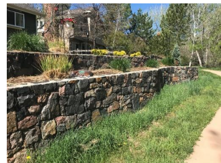
Photo 35: Rock retaining wall (CSFS, 2020)
