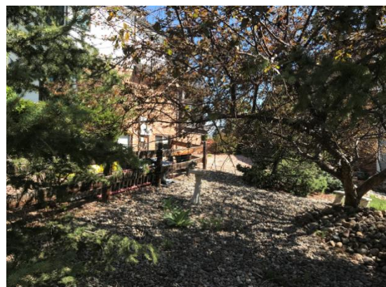
Photo 38: Rock between homes and non-combustible fence along siding (CSFS, 2020)
