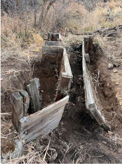
Fall 2023, diverter excavation view to west
